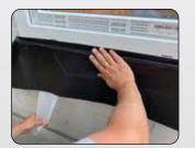
Remove the small protective film (+/- 25 mm) so that a small part of the adhesive appears. This will serve for fixing to the joinery.
