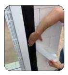
3. Remove the connecting parts of protective foil so that a connection can be made with the structure. Take into account a recommended width of 8 cm on porous substrates (10 cm for the CS-EPDM Easy Foil).
