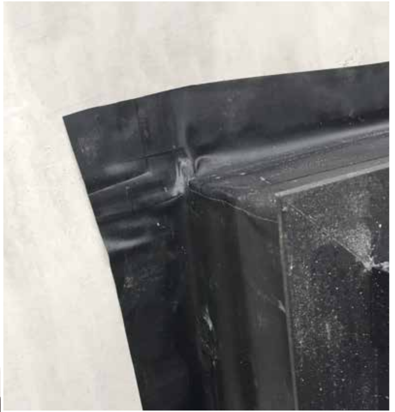
EPDM Window Frame with welded corners
