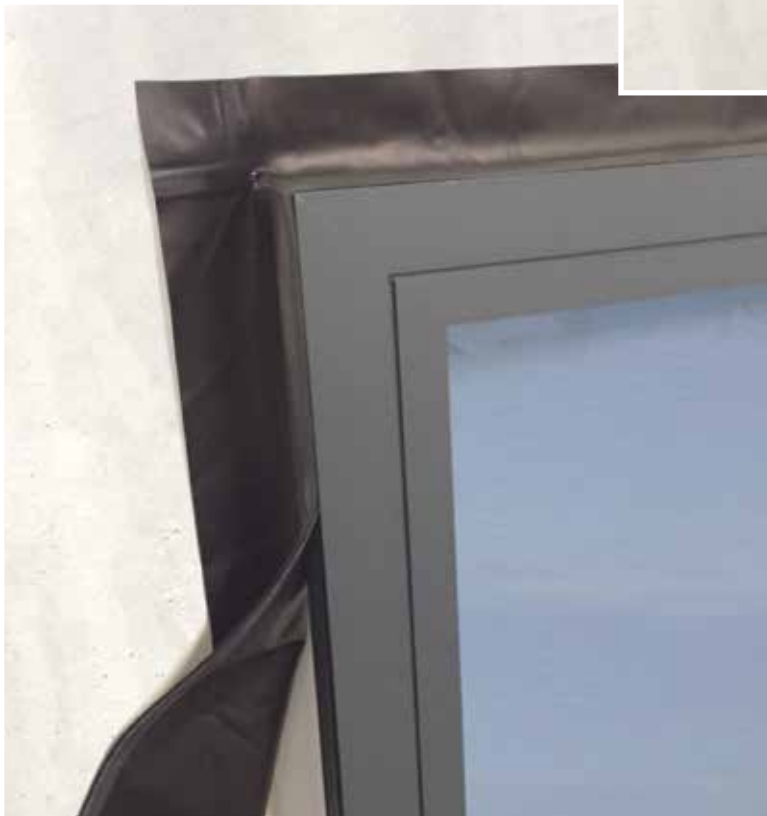
Π-shape EPDM with gasket
