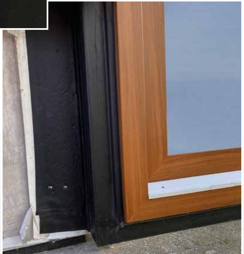
EPDM Window Frame with welded corners
