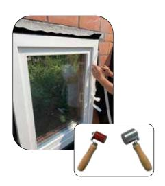
2. Remove the protective film from the butyl adhesive strip and press it onto the joinery. Press on with a hard pressure roller.
