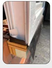
3. Remove the protective film from the butyl adhesive strip and press it onto the joinery. Press with a hard pressure roller. The receptacle (part 1) is now in position.
